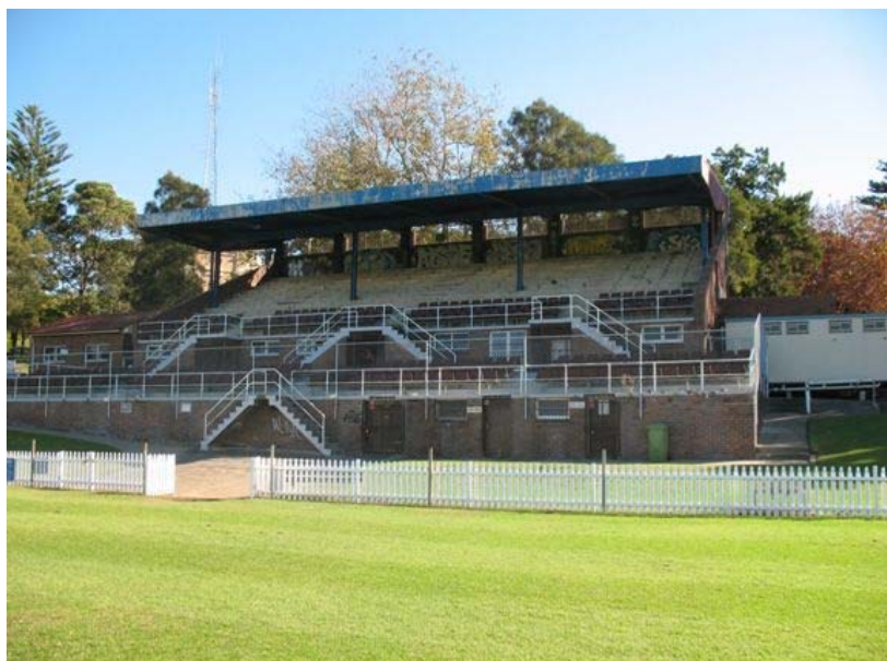
Right: Waverley Pavilion as it is today. The very large referees change room can be seen to the right of the grand stand.
